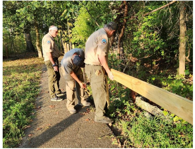
Installing wooden handrails
